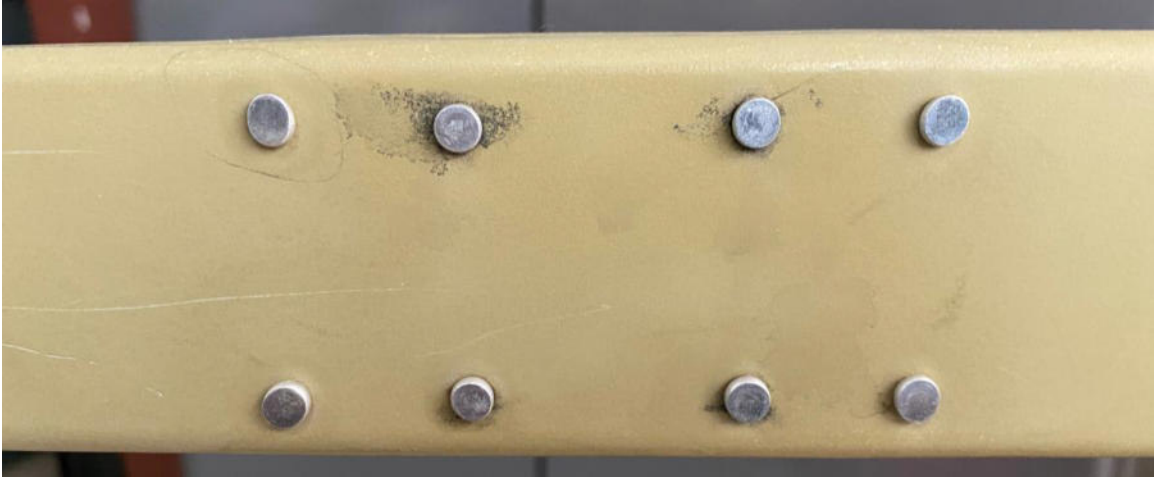
FIGURE 3 - EXAMPLE 2 - CRACK LOCATIONS - FWD SIDE OF SPAR
