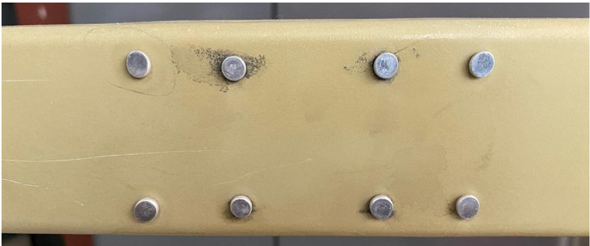
FIGURE 3: EXAMPLE 2 - CRACK LOCATIONS - FWD SIDE OF SPAR
